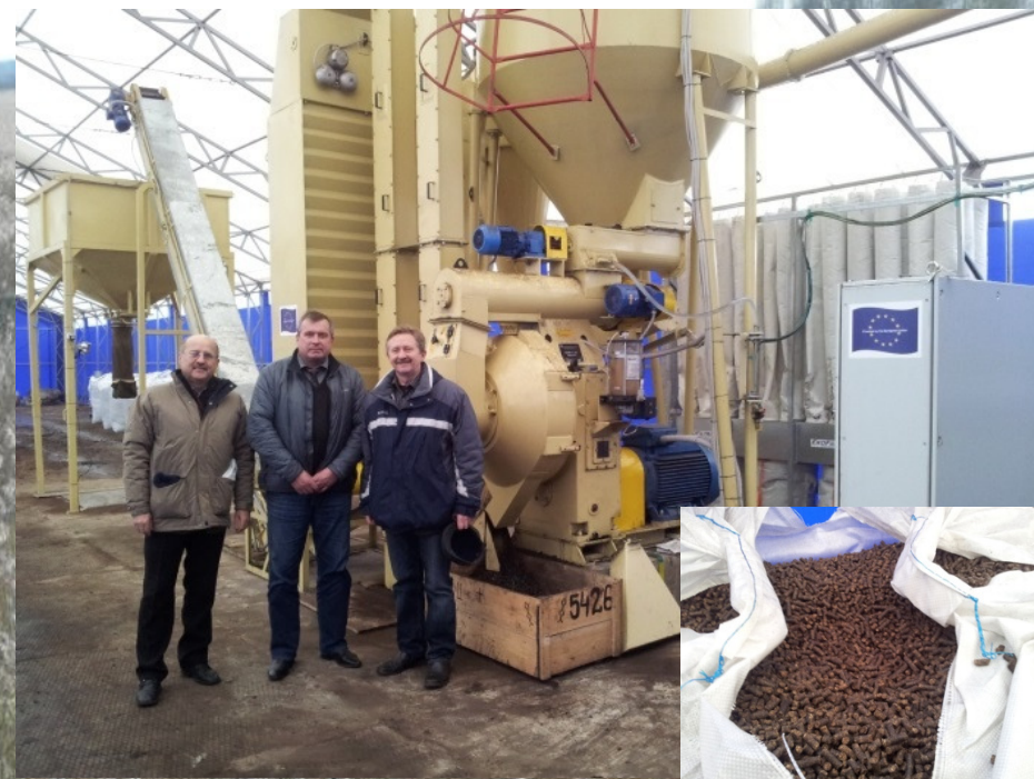
Pellet line for the production of biomass pellets
